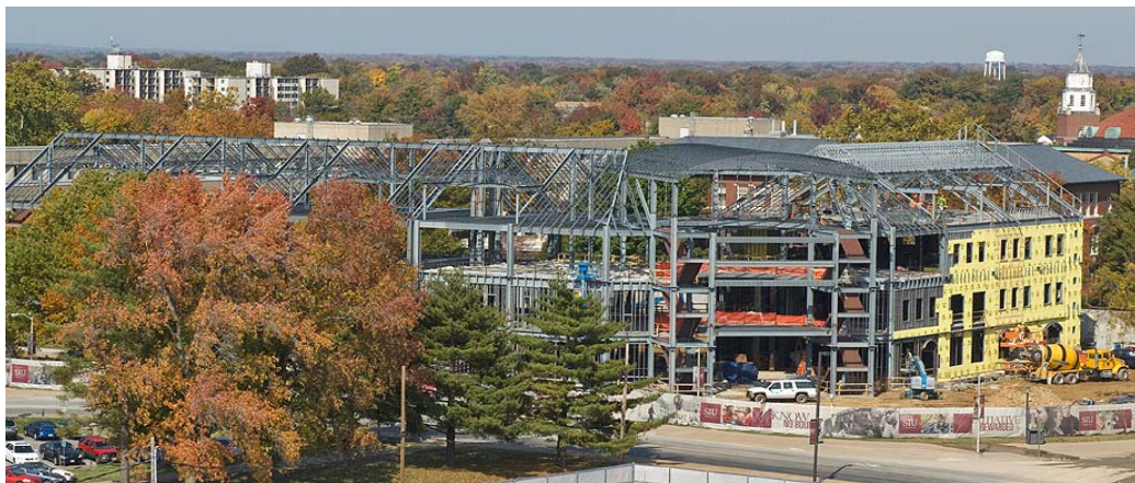
Construction of the new Student Services Building at SIU Carbondale
