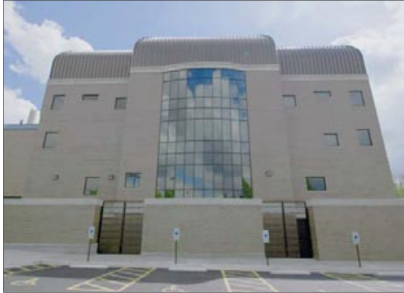
Springfield Combined Laboratory Facility Addition
